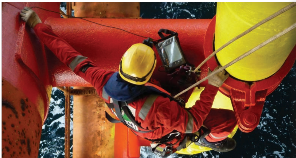
Above: CAN Group's latest contract win will see the company providing ultrasonic inspections as part of structural survey work
